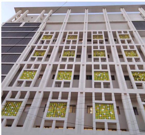
EPS SCREEN HOSPITAL PROJECT
