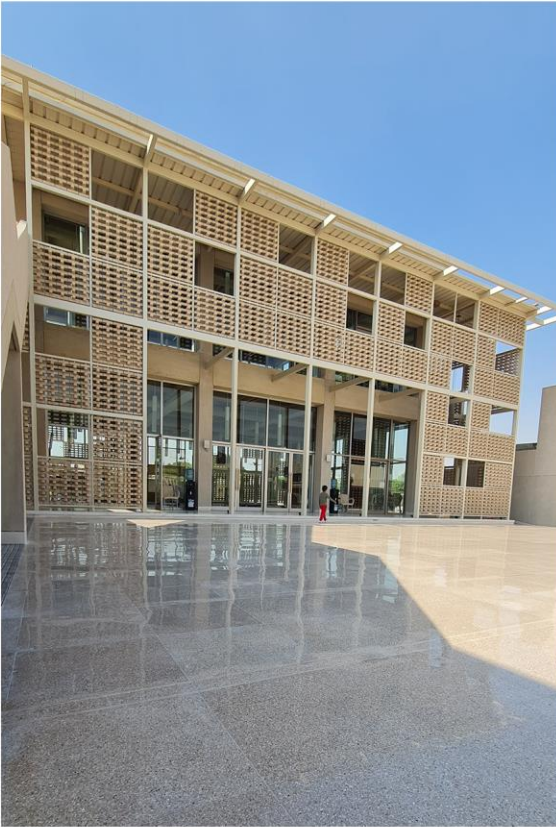
DRY CAST BRICKS AT MASJID
