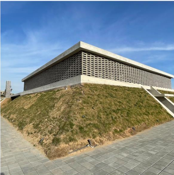
DRY CAST BRICKS AT MASJID
