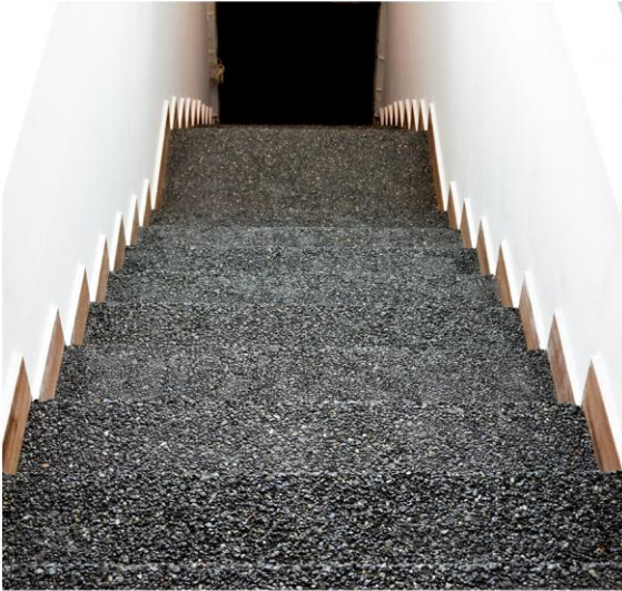
WASH TERRAZZO STEPS AT A PRIVATE OFFICE
